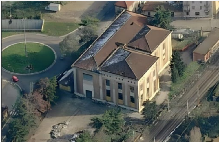
Aerial view of the building
